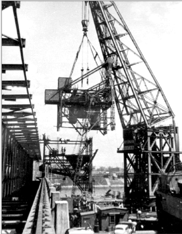
Titan placing a top section (two new Stothert & Pitt gantry cranes) Oct 1954 for bulk sugar in loading at CSR Pyrmont Refinery. Insert shows 4.5 ton grabs discharging Japartit in 1978
